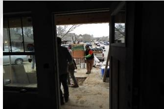
Staging the cabinet bases in the correct alignment per the building plan was critical and following the plan the members began to secure the base cabinets to the walls, providing a solid foundation for the kitchen for many years to come.
