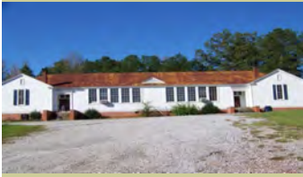
Woodworking Education Center 10544 Hwy 17, Maylene, AL 35114
