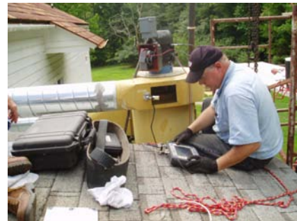
Randy Upton balancing the Dust Collector
